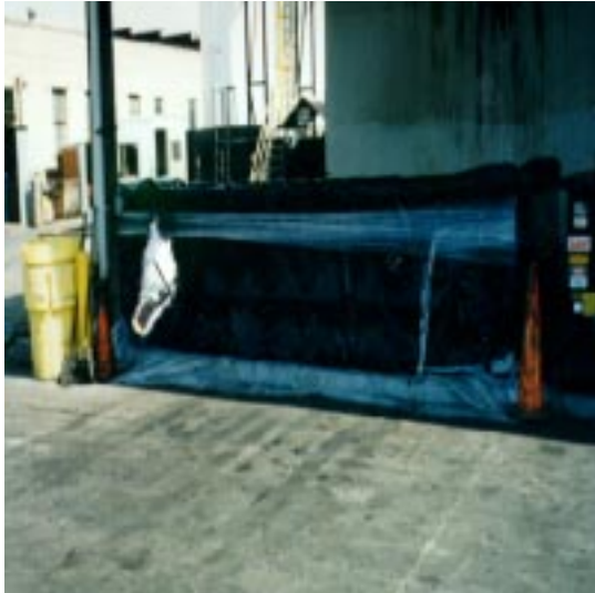
Photograph of a rolloff which contains volatile organic waste. Note that there is no cover on this unit.
